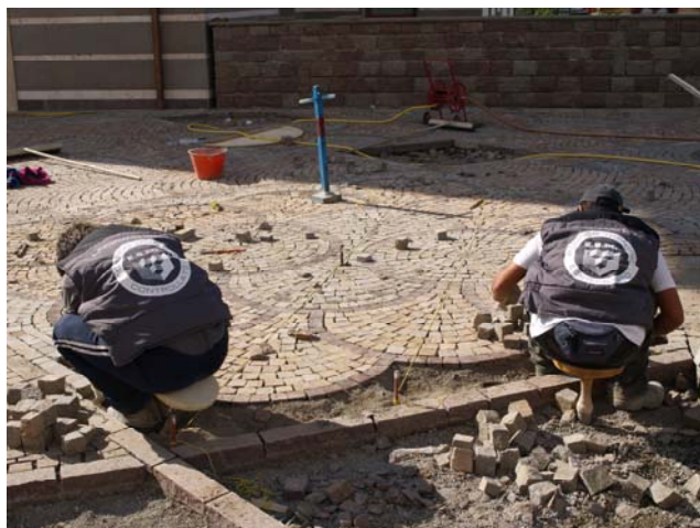
Posa in opera
